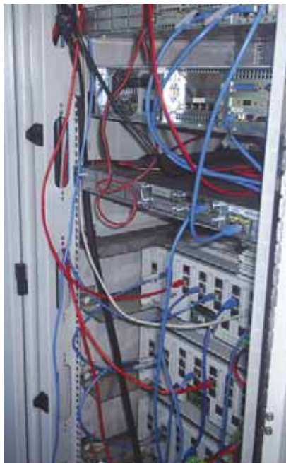
Unstructured base station cable installation
