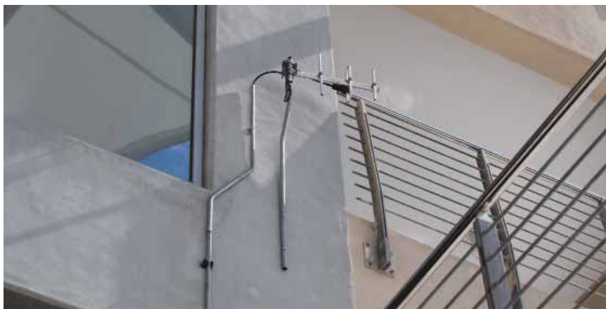
Top left: Repeater installed into one underground tunnel in the Yas Marina Circuit area. Top right: Field strength with the repeater off. Left: An uplink antenna receiving the base station's signal and delivering it to the repeater.
